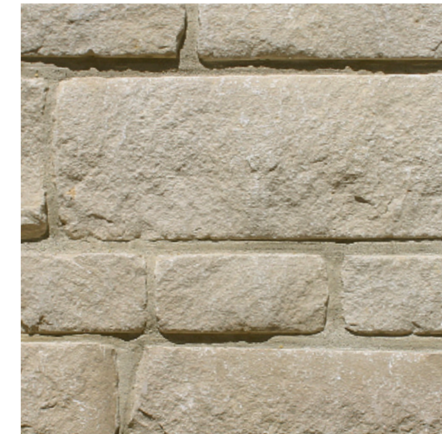
Nadia PILLOWED LEDGE Raked mortar joint
