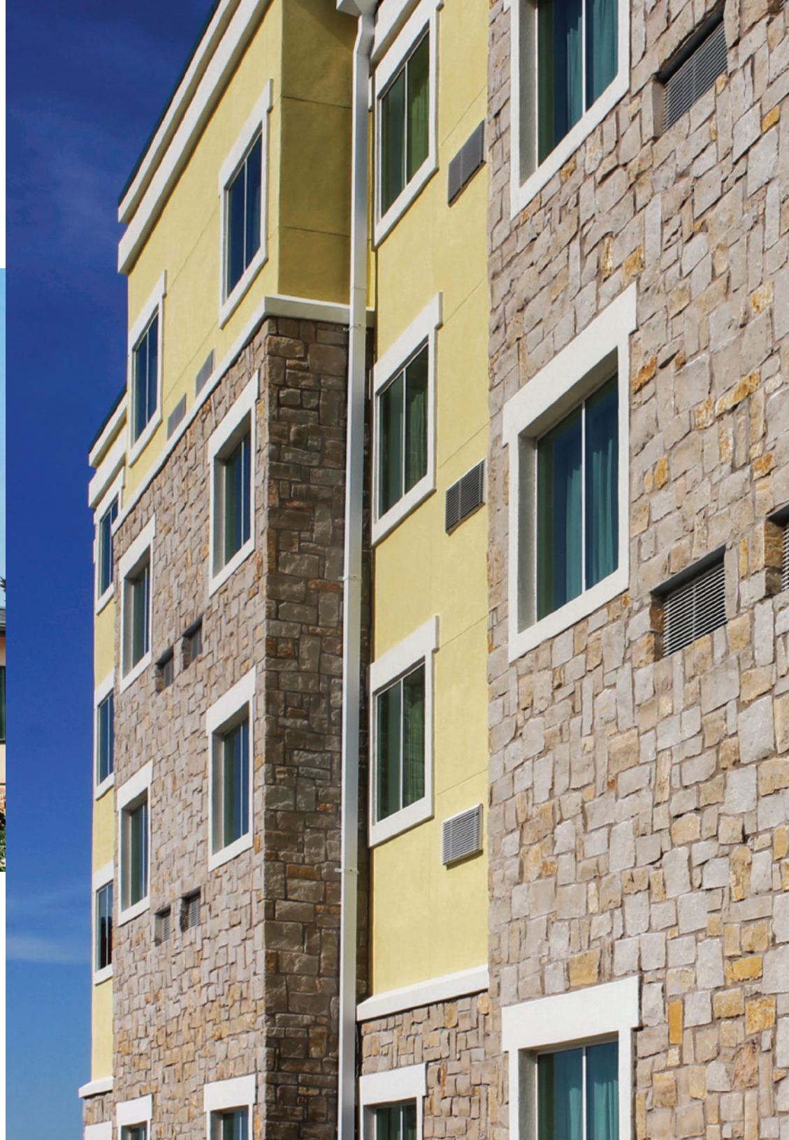
ABOVE: REGENT BUFF RUBBLE INSTALLED STANDARD RAKED JOINT MIDDLE: HONEY BUFF RUBBLE INSTALLED STANDARD RAKED JOINT RIGHT: TUSCAN BLEND RUBBLE INSTALLED FLUSH MORTAR JOINT
