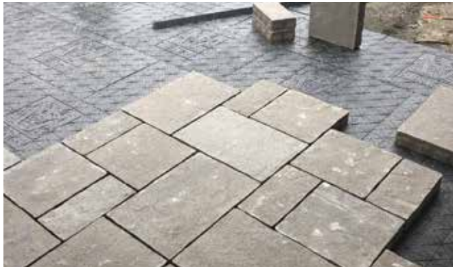
"Much easier and faster to lay the paver down."
